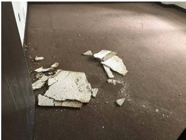
33. View of Unit 119 (vacant).
