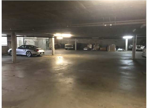
8. View of the subgrade parking area.
