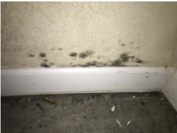
21. View of mold growth in Unit 113 (vacant).
