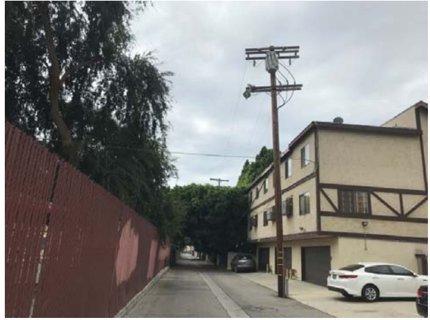
44. View of the adjacent alley to the east and pole-mounted transformer.
