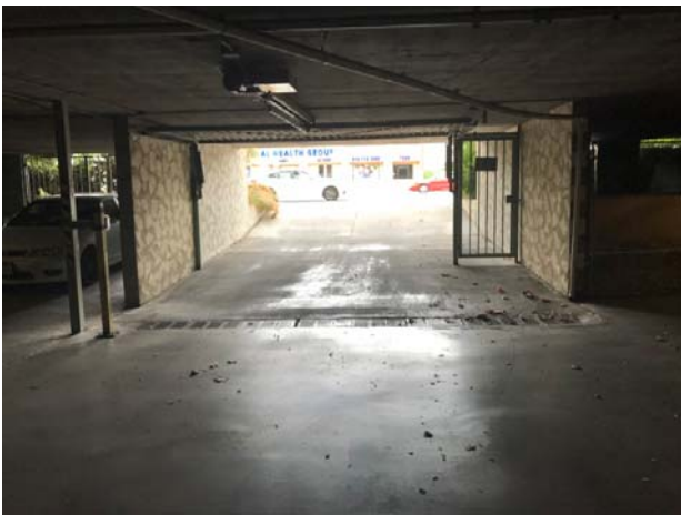
9. View of a subgrade parking entrance and trench drain.
