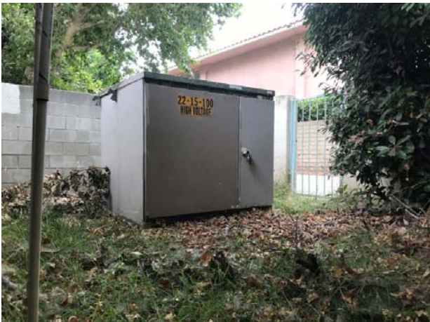
11. View of the pad-mounted transformer situated on the east lawn of the property.
