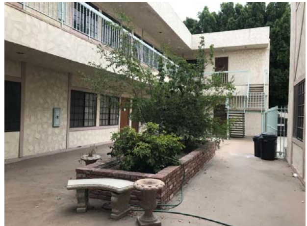
6. View of a patio area.
