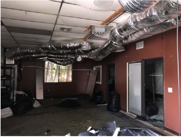
37. View of Unit 209 (vacant, formerly used for marijuana growth operations).
