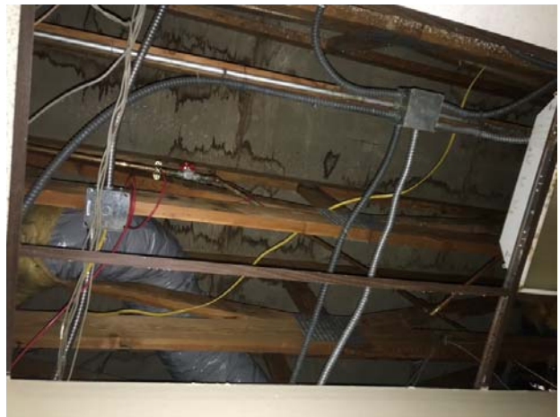
22. View of the water-damaged ceiling.
