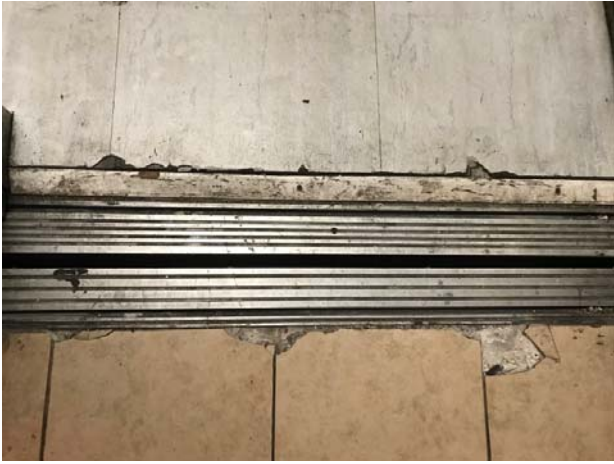
19. View of general cracked and chipped floor tiles.
