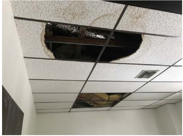
32. View of Unit 117 (vacant).
