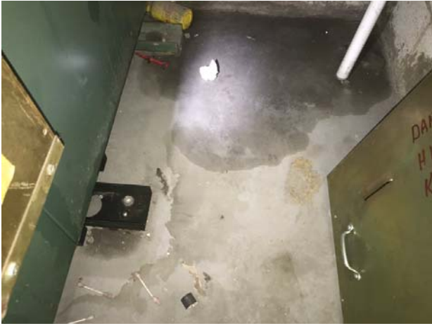
13. View of surficial staining.
