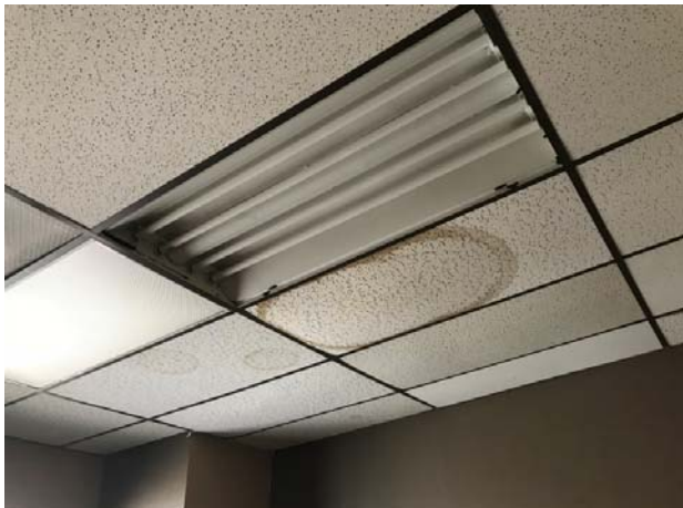
29. View of water-damaged ceiling tiles.
