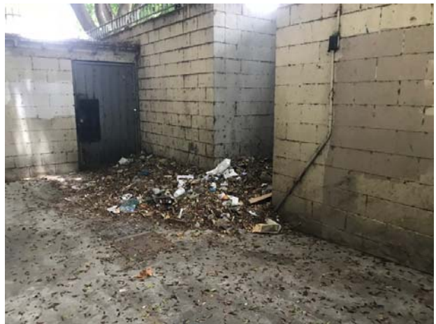
10. View of the vacant subgrade portion of the property situated east of the parking garage.
