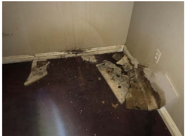
30. View of fallen ceiling tile pieces comprised of dry mold within Unit 219 (vacant).
