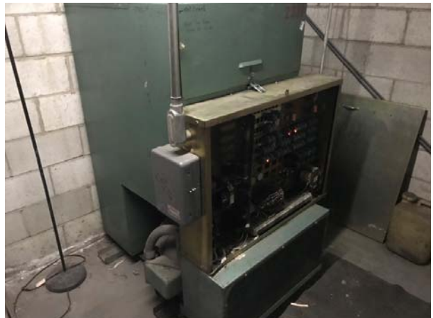
12. View of the elevator motor.
