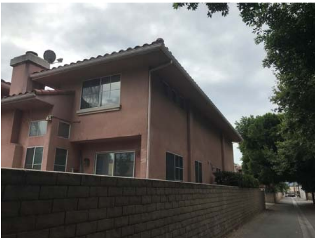
45. View of the adjacent multi-family complex to the east across an alleyway.
