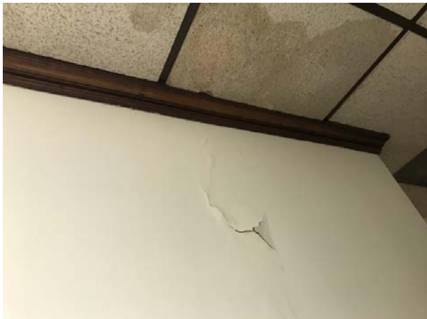
35. View of water-damaged ceiling tiles and dry-wall.
