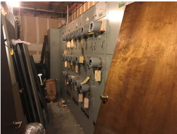
15. View of a general electrical room.
