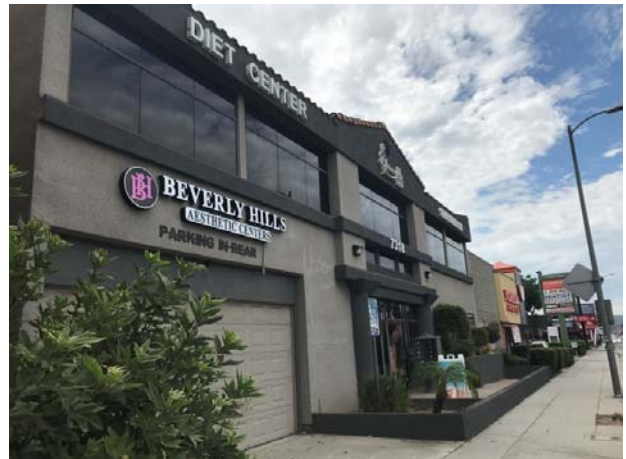
42. View of the adjacent commercial property to the south.
