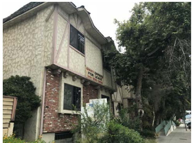
2. View of the front of the subject property from the northwest looking south.
